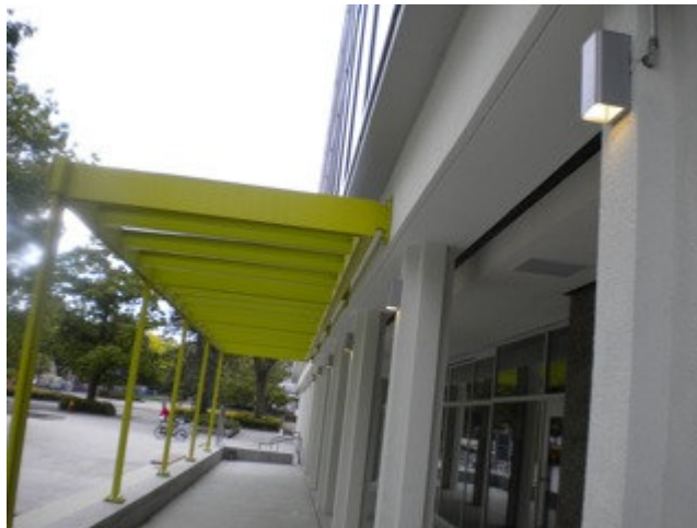
Figure A-5 – Multiple exterior lights operating during midday at recently renovated Sauder School of Business building
