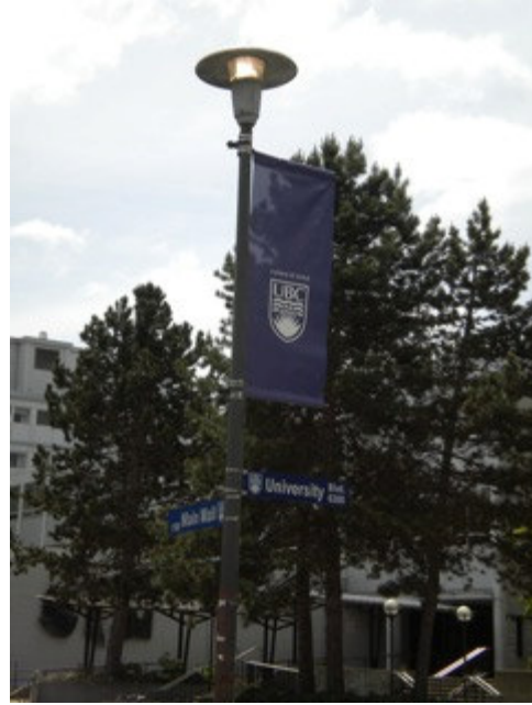
Figure A-4 – Pole lighting operating during day time hours.
