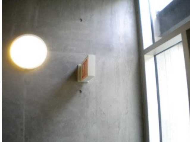
Figure A-6 – Interior lighting operating during daylight hours in a staircase with excellent day-lighting
