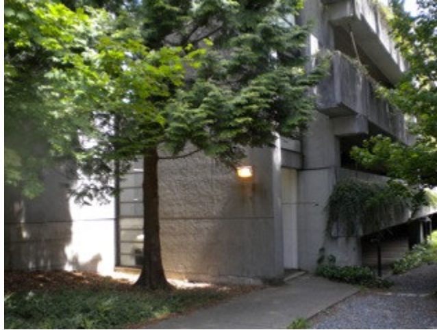
Figure A-1: Exterior light – appears to operate continuously
