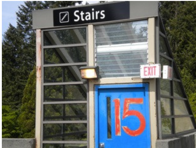
Figure A-2 – Exterior light and interior staircase light at West Parkade operating throughout the day
