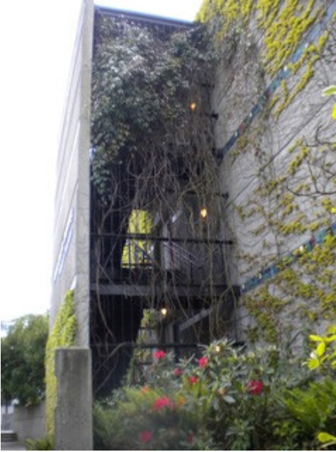
Figure A-3 – Exterior lighting operating during day time hours.
